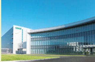
Pharmaceutical plant at the Kanto Factory
