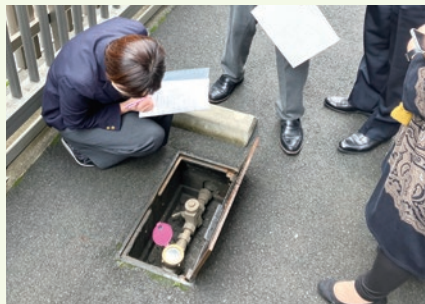
Checking water equipment
