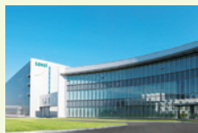
Pharmaceutical plant at the Kanto Factory
