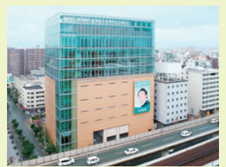
Head Office and Research Laboratories
