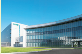
Pharmaceutical plant at the Kanto Factory
