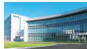
Pharmaceutical plant at the Kanto Factory
